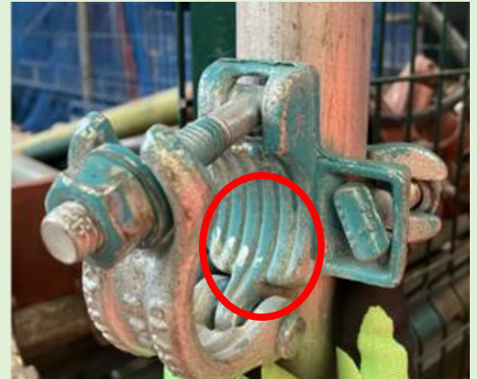
The supplementary Coupler bolt not fully housed (red circle)
