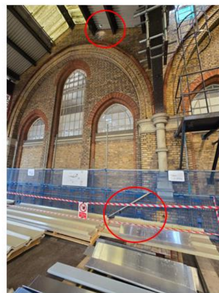
Penetration point (top circle) and scaffold tube landing point on crash deck (bottom circle)
