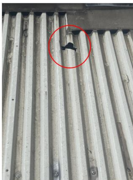
Roof penetration point
