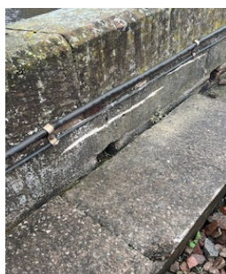
Track Trolleys located in the cess above and the damage caused
